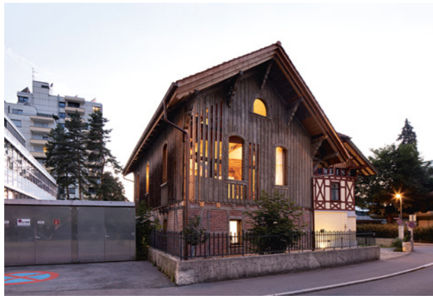
Office and residential building Julia Kick, Julia Kick (2017)
